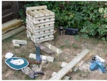
Eighteen 3m half-round pressure-treated fence rails cut into 36cm palings, 10cm dia. Each cleaned off and coated with eco-friendly preservative.
