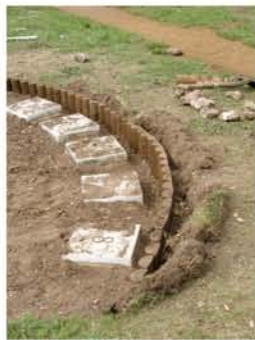
The new logrolls set in, levelled, and back-filled.
