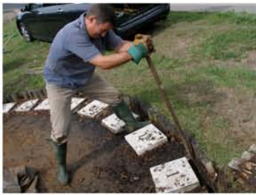
The old rotten logrolls crowbar'd out, and the trench re-dug.
