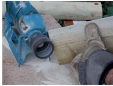
Eighteen 3m half-round pressure-treated fence rails cut into 36cm palings, 10cm dia. Each cleaned off and coated with eco-friendly preservative.
