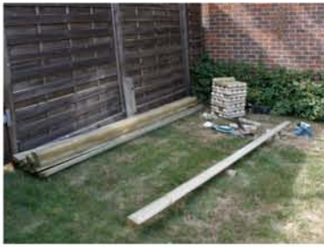
Eighteen 3m half-round pressure-treated fence rails cut into 36cm palings, 10cm dia. Each cleaned off and coated with eco-friendly preservative.
